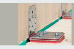
Angle brace with optimal sound insulation
